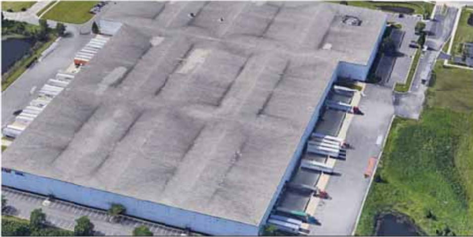
2013 ADDITION: NAPERVILLE, IL
